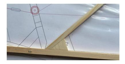
3) Stick the reinforcement plywood with the corresponding number on both sides of the strips.
